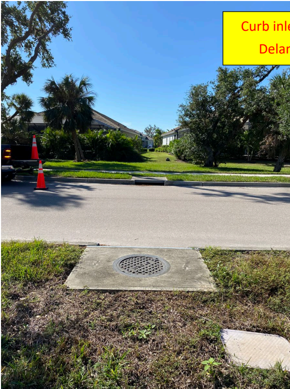
Yard inlet filled with pine straw and debris
