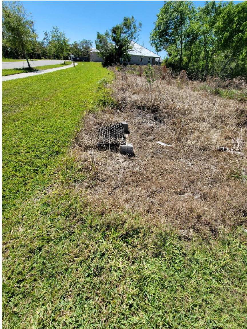
Control Structure - A-2
