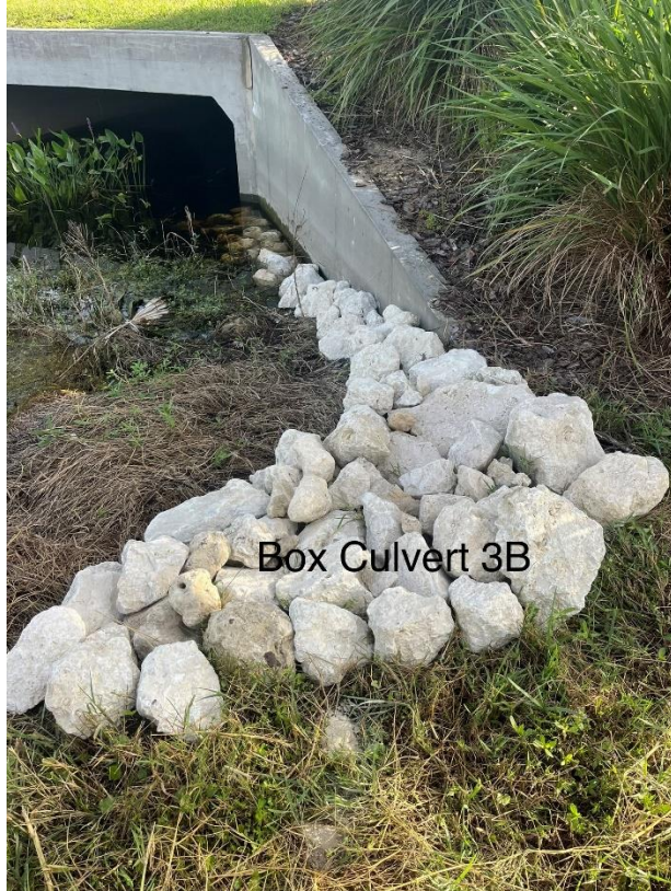
Box Culvert 3B
