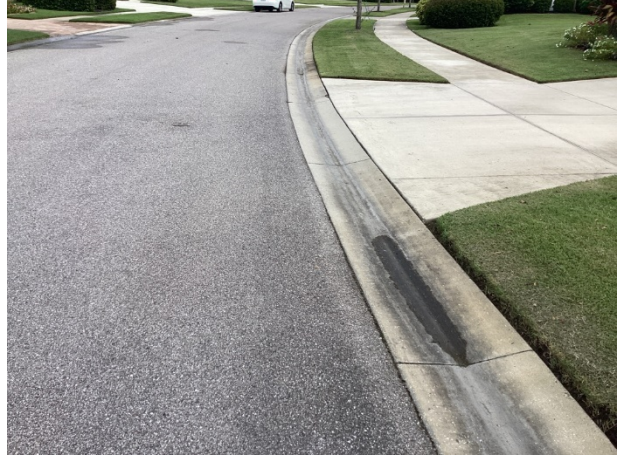
Concrete gutter
