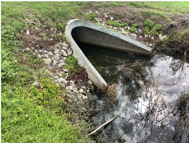
Culvert overview – North Clubhouse
