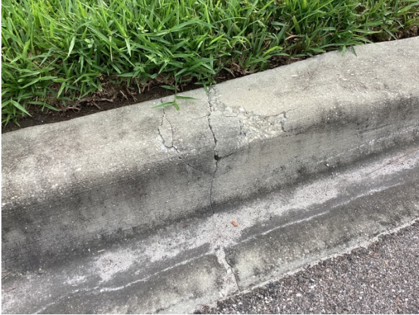
Concrete spalls
