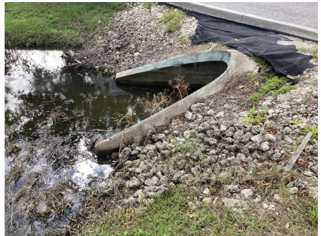
Culvert overview – North Clubhouse
