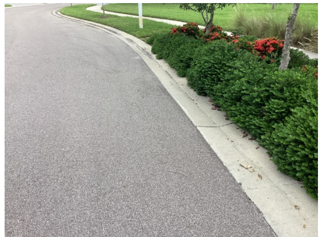
Concrete gutter
