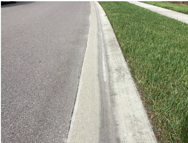
Concrete gutter
