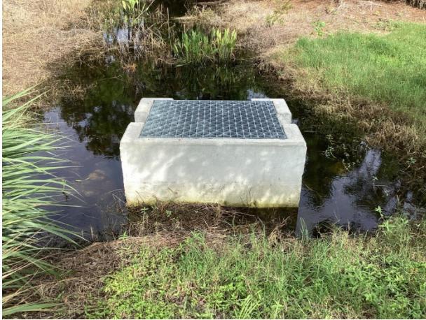
Control structure overview – South Clubhouse
