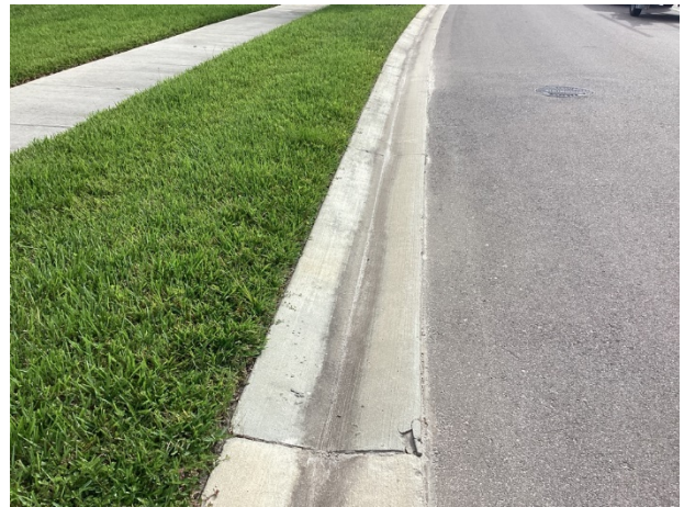
Concrete gutter
