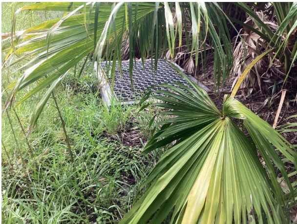
Control structure overview – Aucilla Dr.
