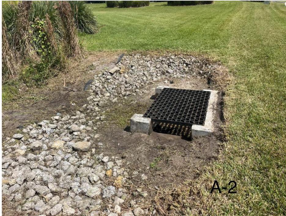
Control Structure A-2
