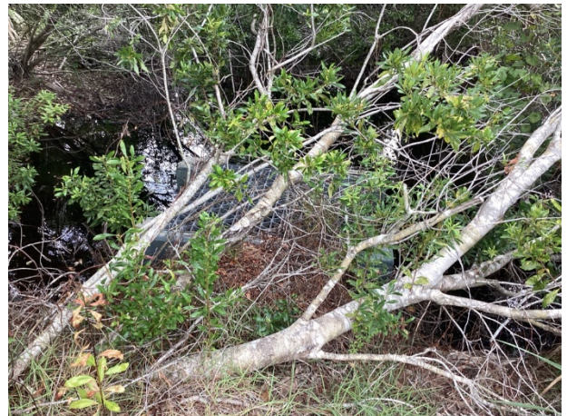
Control structure with debris – Sagewood Dr.
