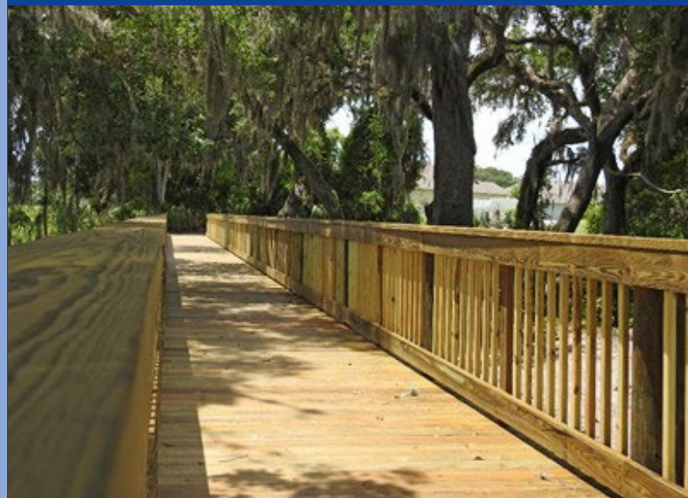
Pedestrian Boardwalk at Oak Creek CDD
