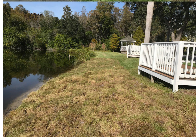
Pond Restoration at Westchase CDD
