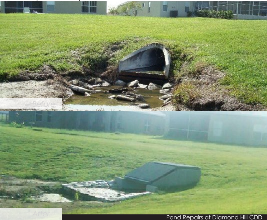
Pond Repairs at Diamond Hill CDD
