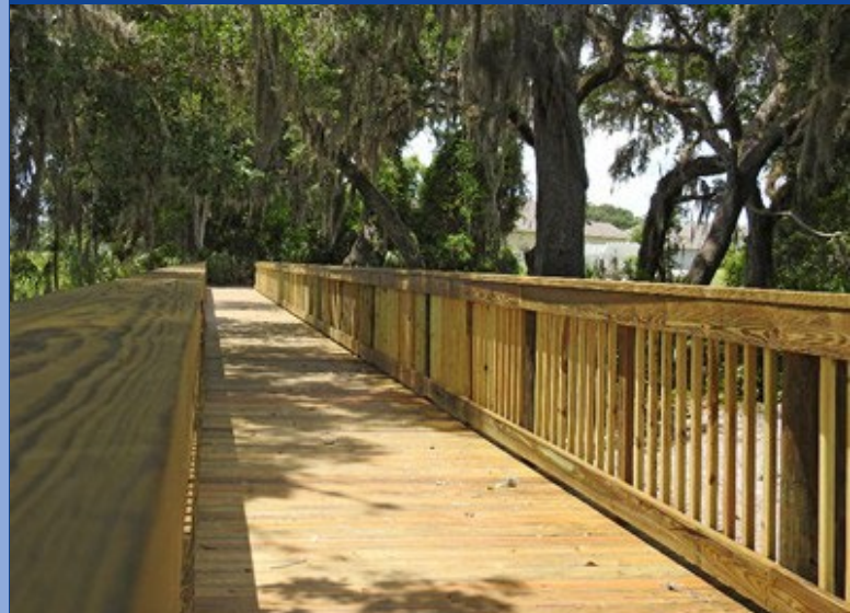
Pedestrian Boardwalk at Oak Creek CDD
