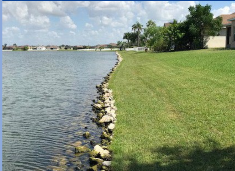
Pond Bank Restoration at Mira Lago CDD
