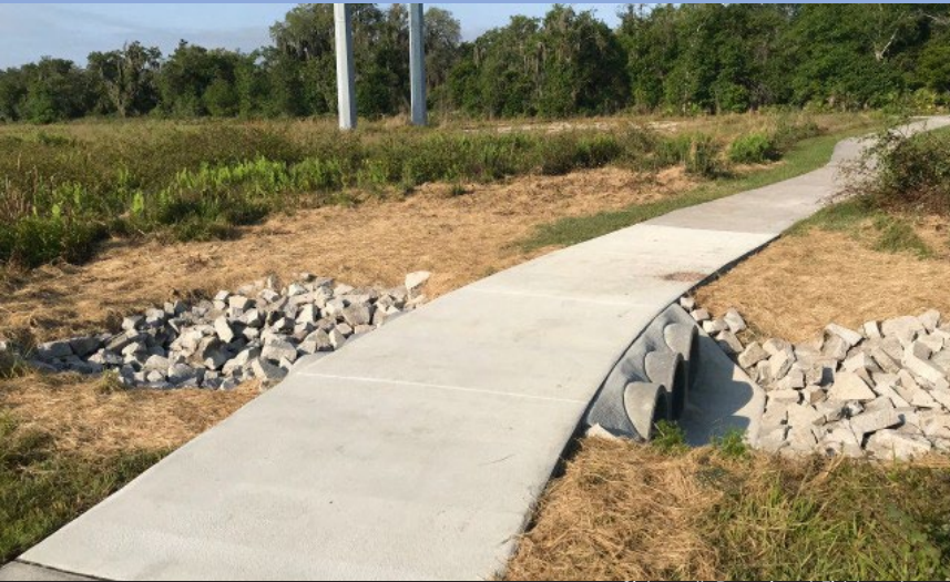
Sidewalk Repairs at Fishhawk Ranch CDD
