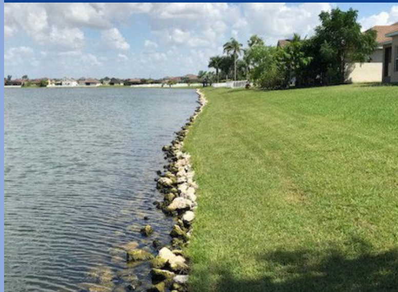
Pond Bank Restoration at Mira Lago CDD
