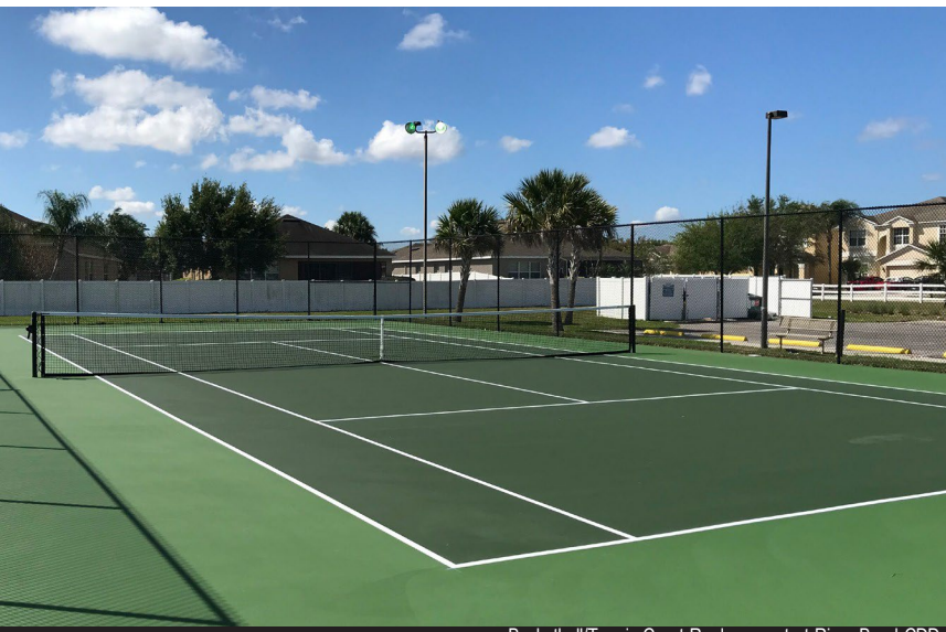
Basketball/Tennis Court Replacement at River Bend CDD
