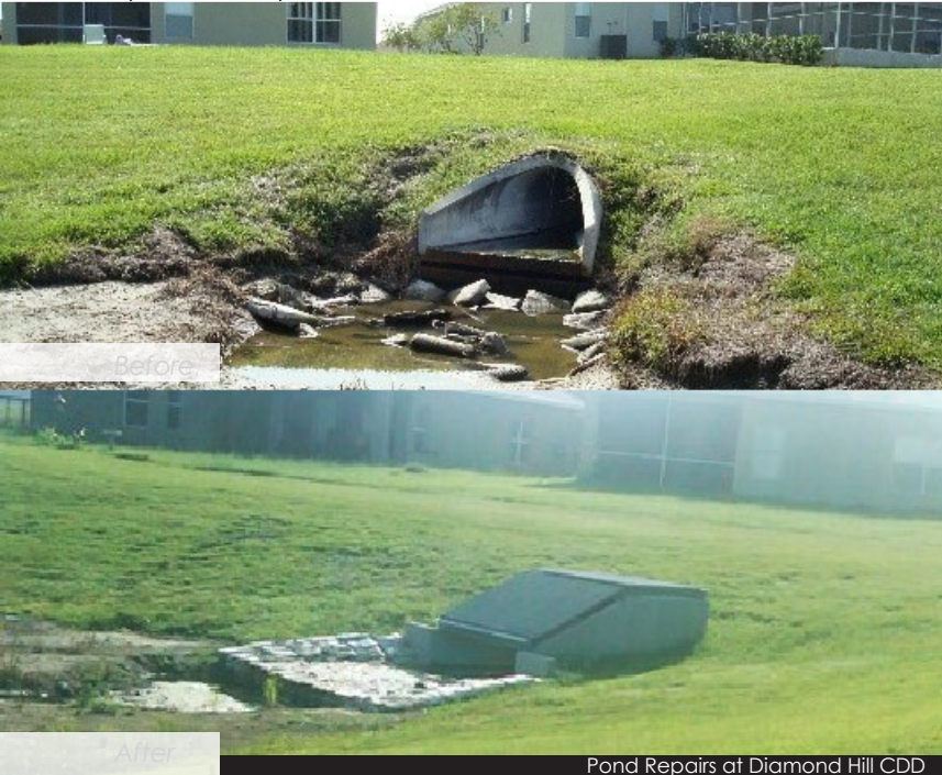
Pond Repairs at Diamond Hill CDD
